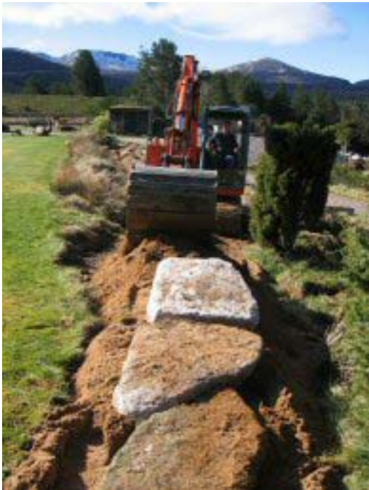
Positioning rocks using the digger
