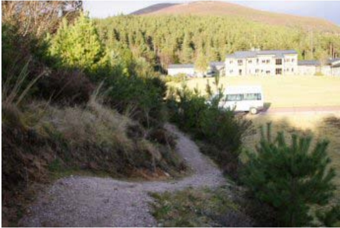
Left: Exit trail from the range showing full bench cut technique
