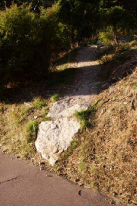
Rock armouring on trail exit to biathlon track
