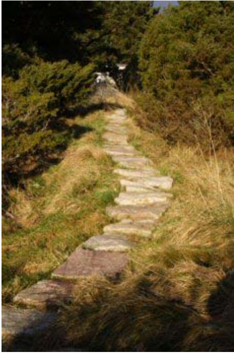
Above left: Raised bench / rock armouring construction
